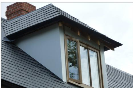
White 9016 3mm Alupanel has been used as the Dormer cheeks on this building. It acts as an impressive weather shield and also provides an element of sound proofing and insulation. The panel has been cut to size
